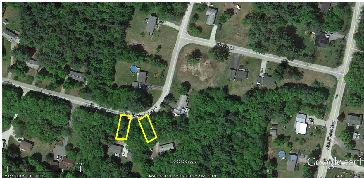
Figure 19. Two compromised culverts conveying stormwater under private drives on Cedarwood Terrace (highlighted in yellow).
