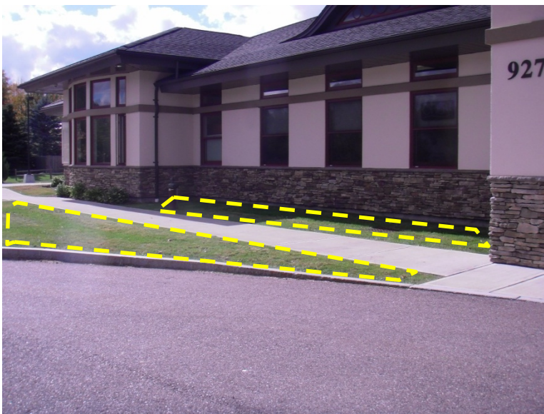
Figure 2. Example of area where roof runoff could be routed to a rain garden.
