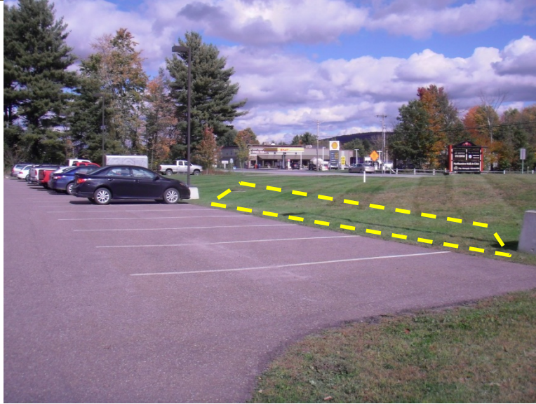
Figure 3. Catch basin is located beneath red pickup truck in the photo. Stormwater from half of parking lot could be routed to lawn area shown right half of photo.
