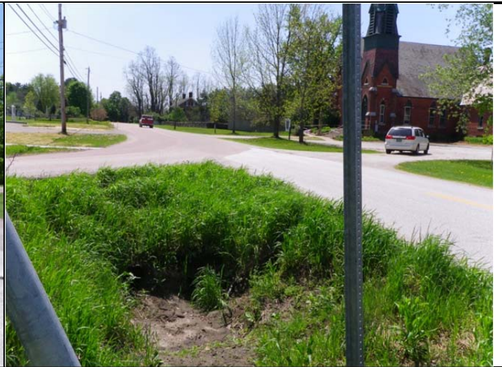
Photo 2. Sediment build up in the "Y" median
